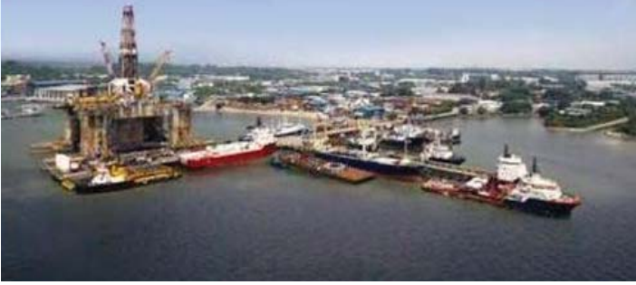
Marine Jetty and Offshore Support Base, Loyang Singapore
